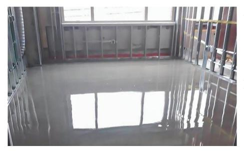
Extremely high moisture levels in the hospital's flooring substrate were a serious problem. Because the renovation project was on a fast track to completion, the Ardex MC Rapid moisture control system, which dries in as little as four hours, was used to reduce moisture levels.
