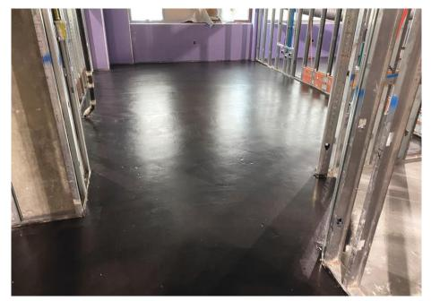
The original flooring at Grady Memorial Hospital dates back to 1892 and renovations and additions over time created a variety of issues that needed to be addressed. As a first step, Ardex K 13 self-leveling underlayment was used to level and smooth the substrate to create a surface that would handle any type of resilient flooring.
